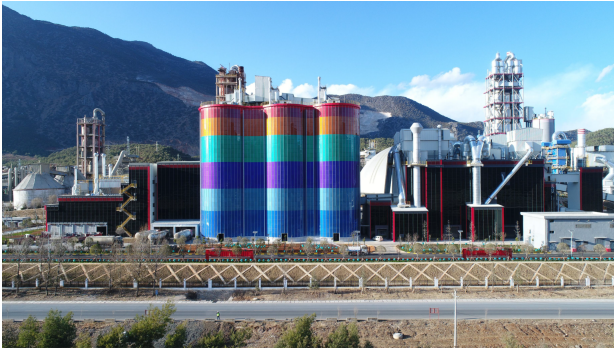
Fig. 7. Status Photo of the Industrial Building Facade after Renovation
