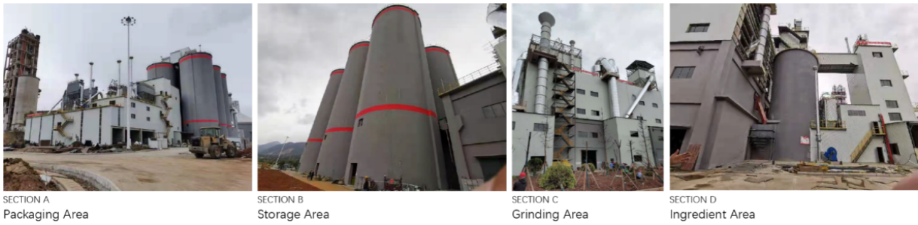
Fig.2. Status of building facade
