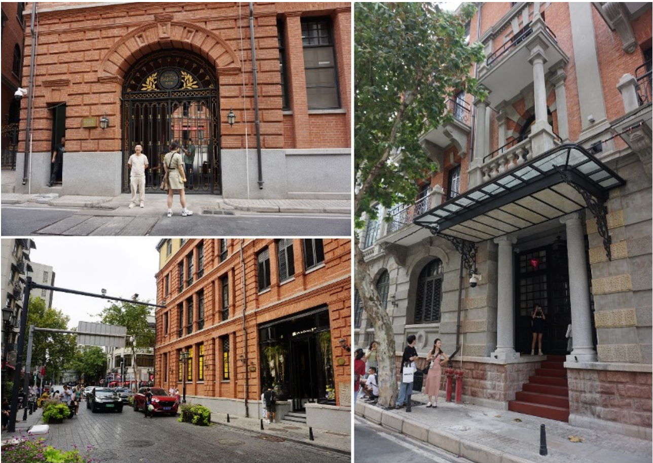
Fig. 5. Details of the renovated building facade
