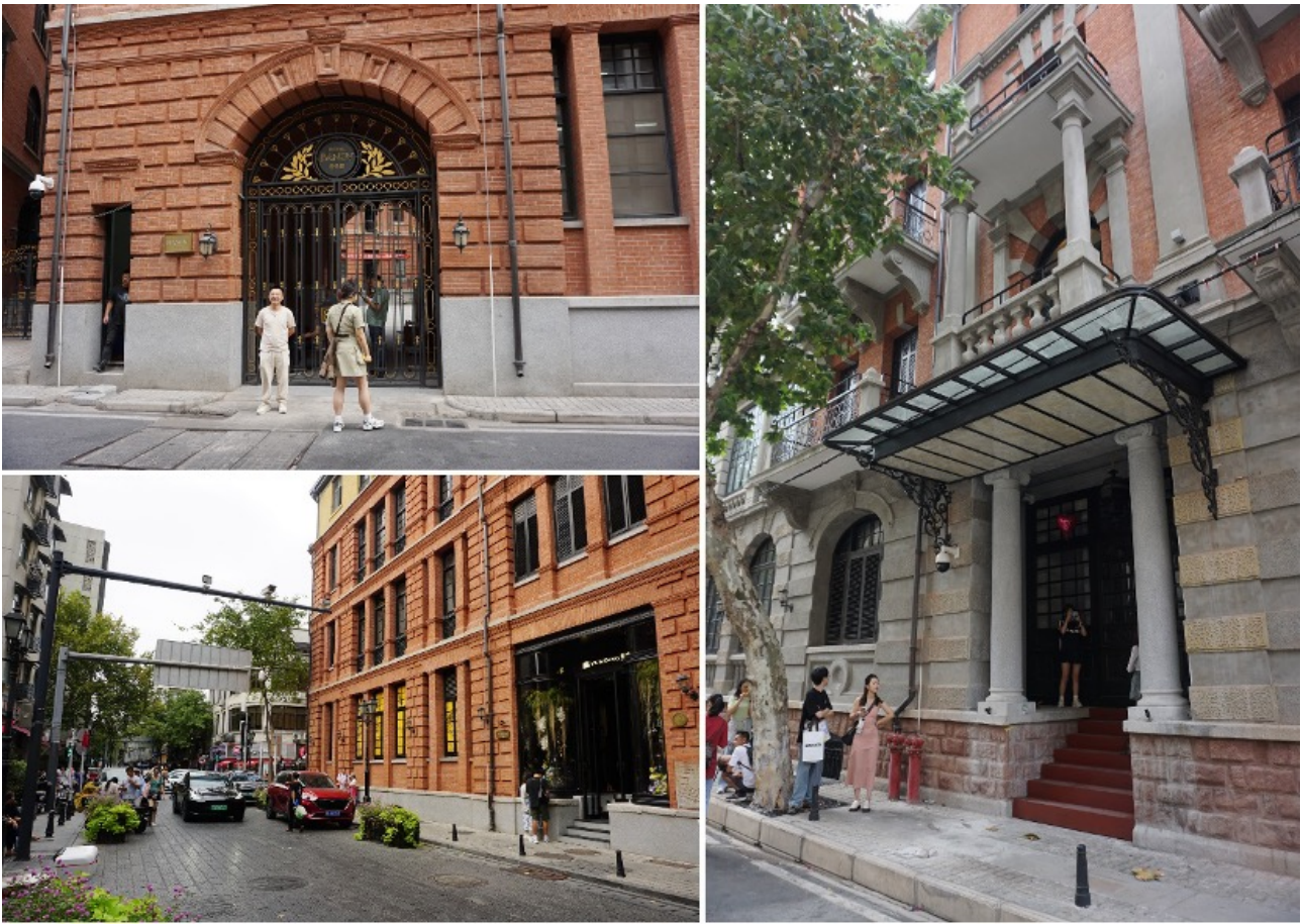
Fig. 5. Details of the renovated building facade
